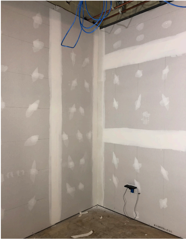
Figure 2. Documentation of on-site observation of gypsum wallboard installation and finishing shows varying board orientations and finishing at seams, corners, and screw locations. Image by Author.
