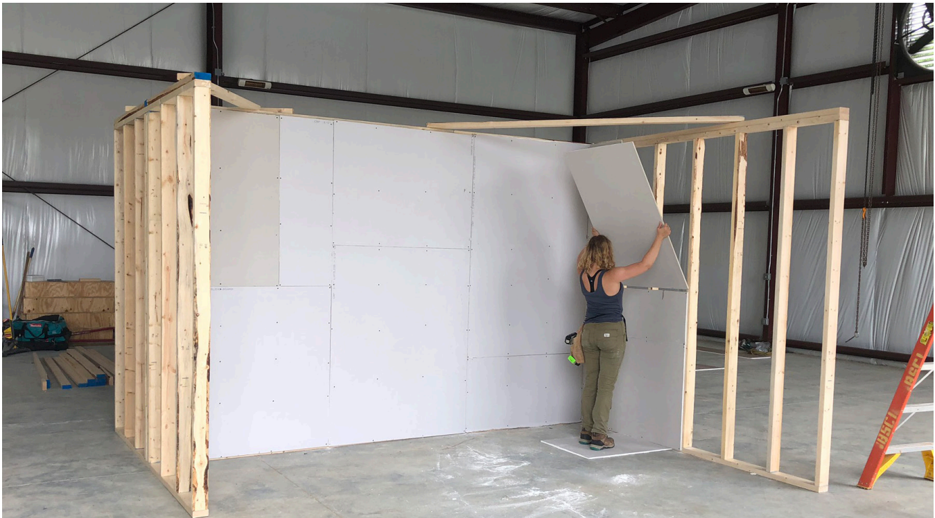
Figure 3. Full scale framing mock-up used to test various module sizes of gypsum wallboard. Image by Author.
